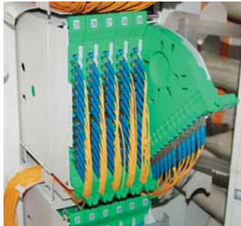
Detail of terminal frame
